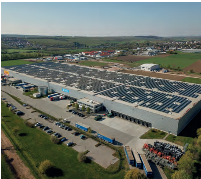
Frankfurt Bodenheim, Germany Photo for illustrative purposes only
